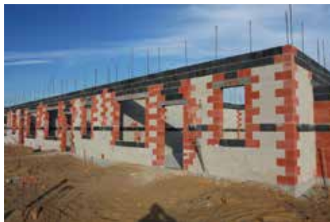
▼ Above – Cat5 Block homes under construction
